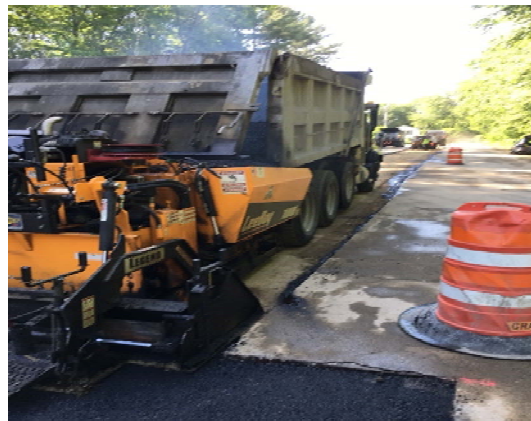
Begin trench repair on North East Blvd.
