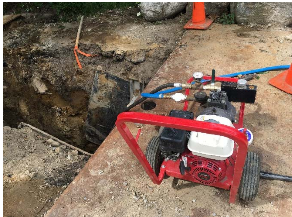
Pressure-Leakage testing all installed Sewer Mains
