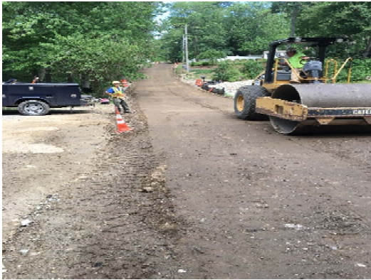
Finished fine grading of gravels
