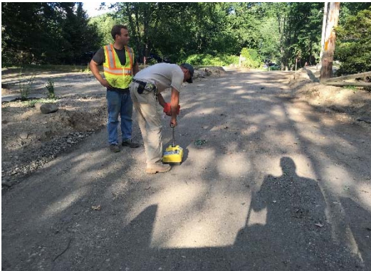
Compaction tested gravels prior to paving
