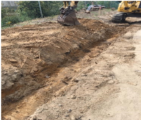
Begin shaping drain swale at #72 S. Shore Rd
