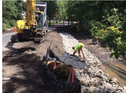
Construction of drain swale at #19 S. Shore
