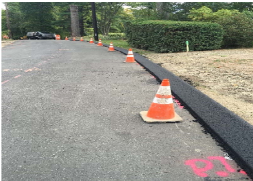
Installed Bituminous Curbing
