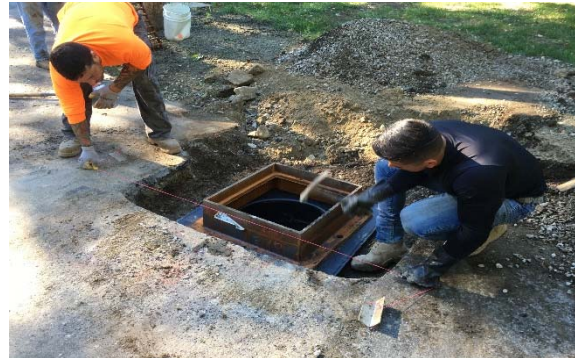
Raised all drainage and sewer castings
