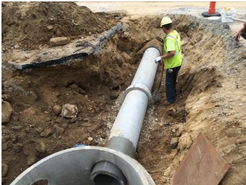
Installation of Drainage Pipe along Main Street
