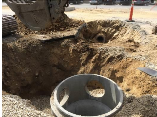
Installation of Drainage Manhole on Main Street
