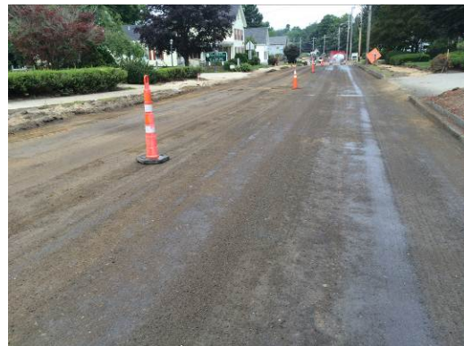
Pavement Removal Operations Along Main Street
