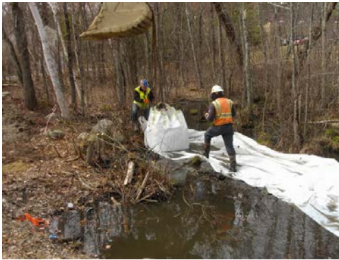
Installation of Erosion Control Measures
