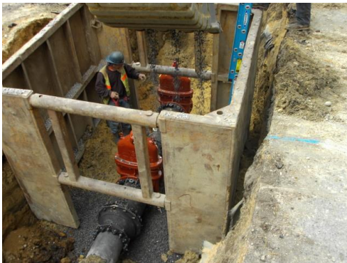
Installation of 16" water main heading North from the Water Treatment Facility to the limit of work
