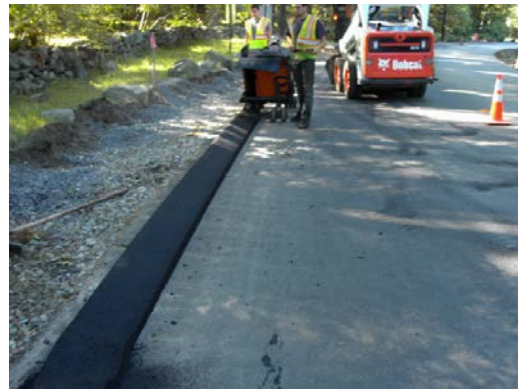
Installing Bituminous Curb
