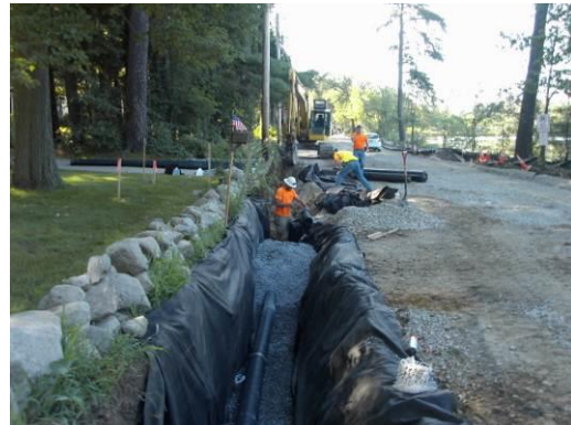
Installing Underdrain
