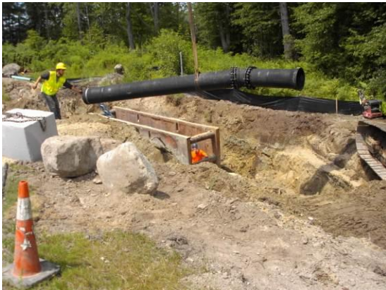
Continued Water Main Installation to the Water Treatment Plant
