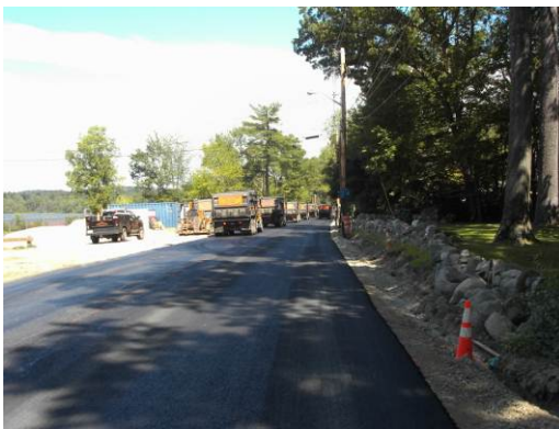
Base and Binder Course Paving Operations
