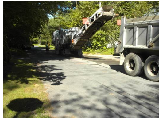
Milling Roadway at Limits of Work
