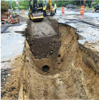
5/28/2014 – Drainage installation near Lowell Road (NH Route 38)
