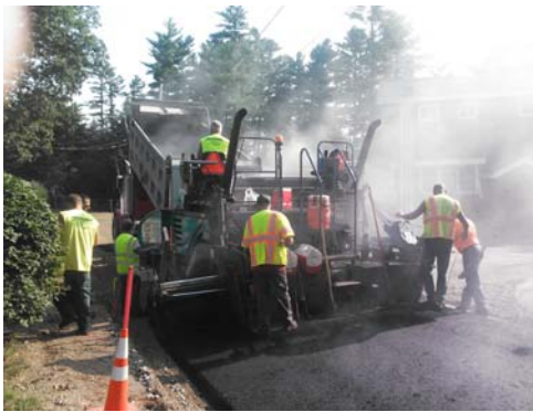
7/18/14 – Paving 1 st layer of pavement on Field Ave near #9.
