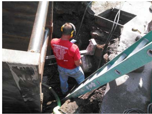
7/23/14 – Coring hole in the side of a drainage structure to begin a new drain pipe run at the intersection of Independence Dr. and N. Main St.
