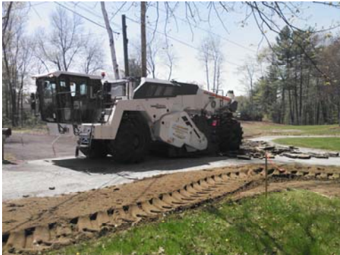
5/12/14 – Reclaimer is grinding up Therirualt Ave.
