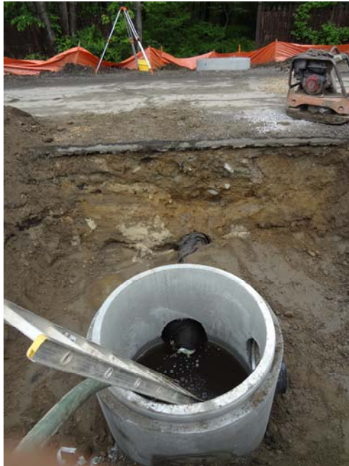
Drain structure installation at #38 Pond Street
