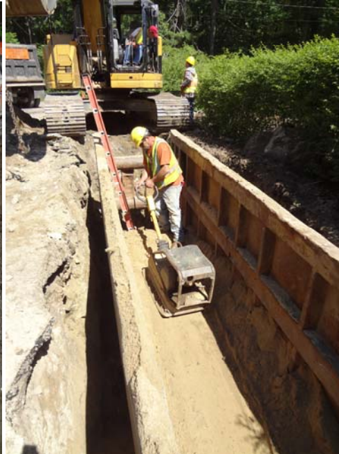
Water main work along Pond Street adjacent to address #34.
