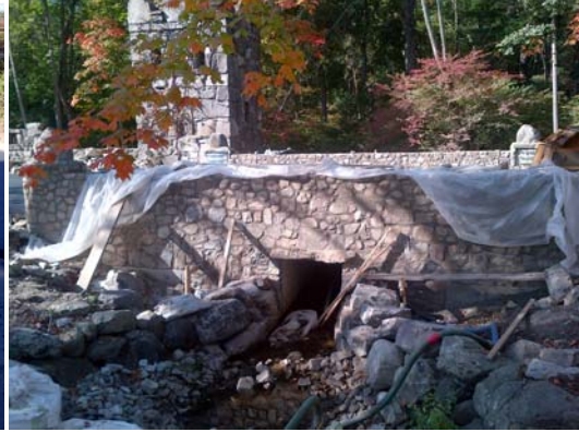
Stone veneer nearly complete on the new box culvert near #70 Pond St
