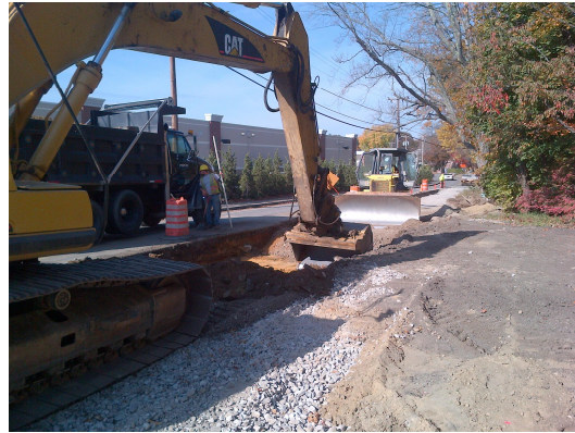
Excavation and replacement of gravels at Hampshire Road and Sand Hill Road Intersection
