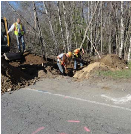
5/2/2013 – Test Pit Excavation in the Vicinity of the Triple Culverts adjacent to #85 & #91 Stiles Driveway.
