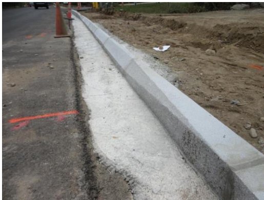
8/29/2013 – Granite Curbing Installation
