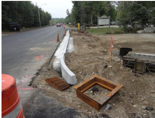
8/29/2013 – Frame and Grate Installation
