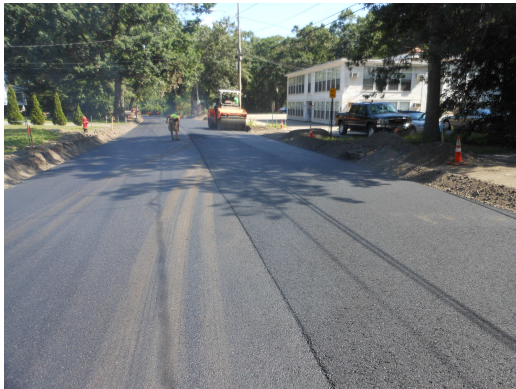
7/2/2012 – Installation of Base Course Pavement near the Foss School
