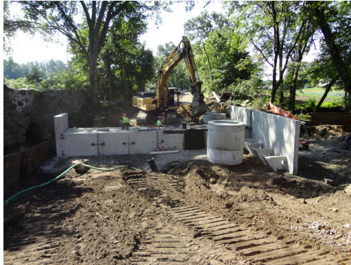
8/21/2012 – Box Culvert Under Construction
