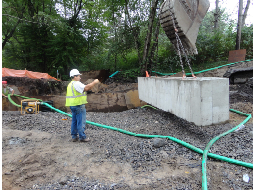
8/18/2012 – First Box Culvert Footing Being Placed
