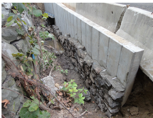
09/18/2012 – Stone Veneer Installation at Box Culvert
