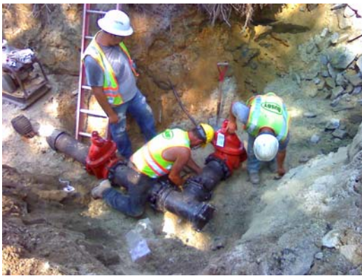
8/9/12 – Water main installation on Pumping Station Road at Jill Road.
