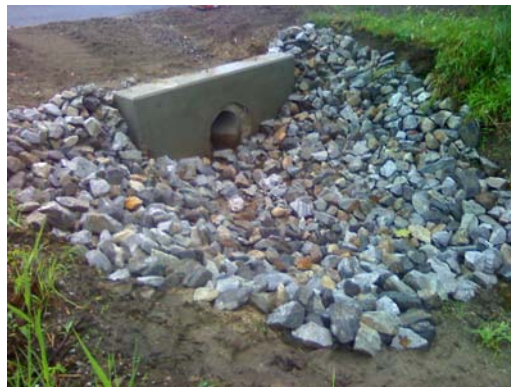
8/7/12 – Headwall installation on Pumping Station near #20.
