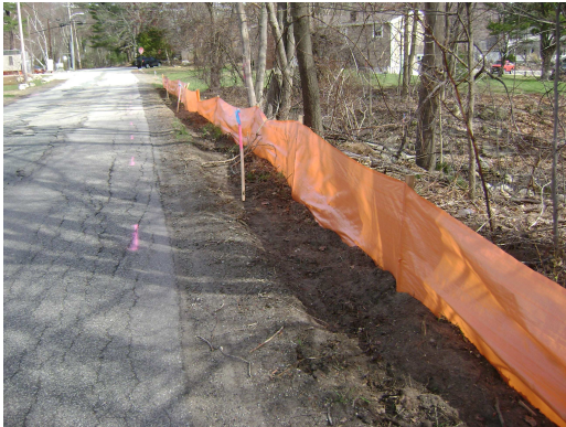
4/21/2011 – Silt Fence Installation Near Pelham Road
