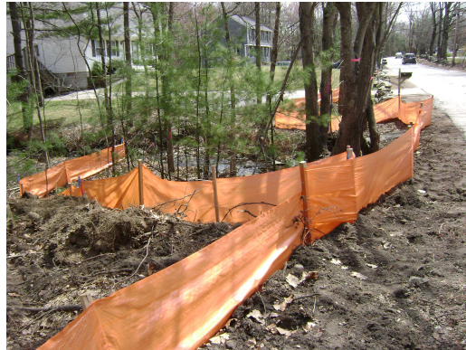
4/21/2011 – Silt Fence Installation Near Cindy Avenue
