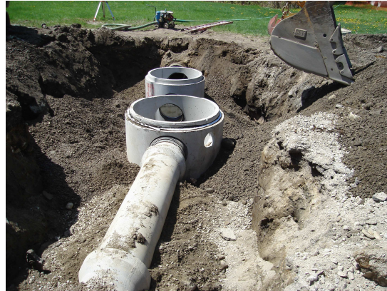
5/05/2011 – Catch Basin Installation On Brady Avenue
