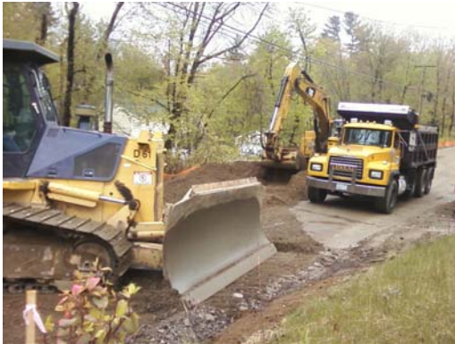
5/2/2012 – Removal of reclaimed material and preparation of roadbed adjacent to #61 Brookdale.
