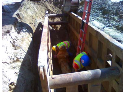
4/25/2012 – Water main relocation adjacent to Northeastern Blvd
