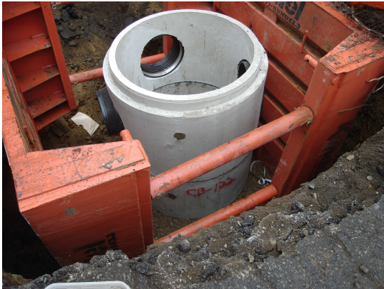
5/11/2011 – Catch Basin Installation with Structure Box On Brady Avenue
