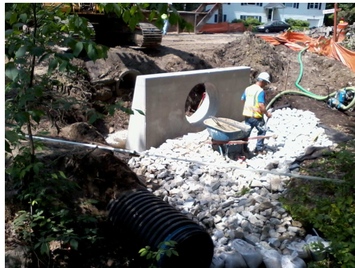
6/8/2011 – Headwall with Stone Apron at the 36" Culvert on Brady Avenue
