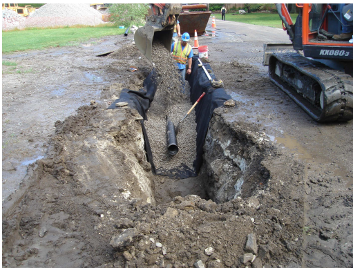
5/25/2011 – Underdrain Installation on Brady Avenue Near Pelham Road
