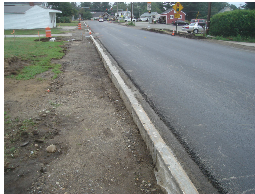
8/10/2011 – Curbing Installation Along Cross Street near Harry's Barber Shop
