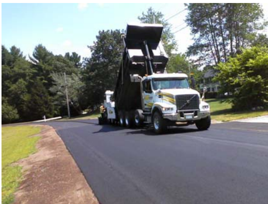
7/19/2011 – Wearing Course paving application near #24 Lisette Drive.
