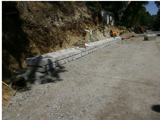
8/20/2010 – Beginning of Retaining Wall Construction near #10 Cluff Road
