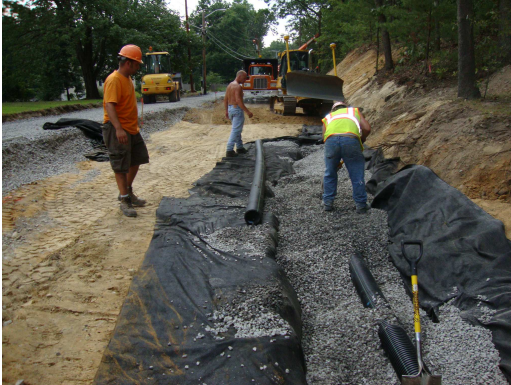
8/10/2010 – Underdrain Installation Near #13 Cluff Road
