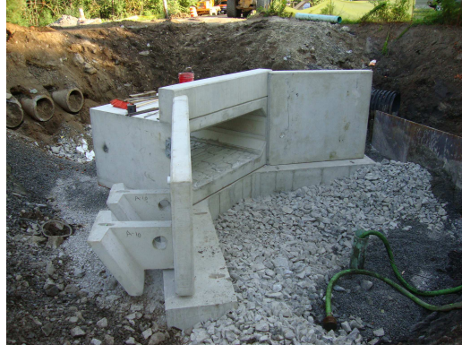
8/11/2010 – Start of Box Culvert Installation
